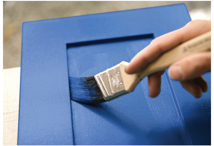
Using a nylon/polyester paintbrush, work from top to bottom, then in full strokes with the grain.
